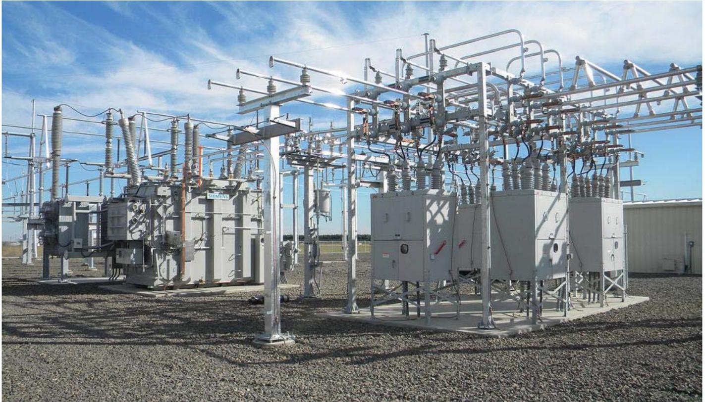
*The ultimate build-out of the new Cloud View substation contains a 230-kV H-bus rated for 3000 A; three sets of transformers, each including a 230-kV live-tank breaker; a 41-MVA 230 x 115/13.8-kV transformer; and a six-bay distribution structure.*
