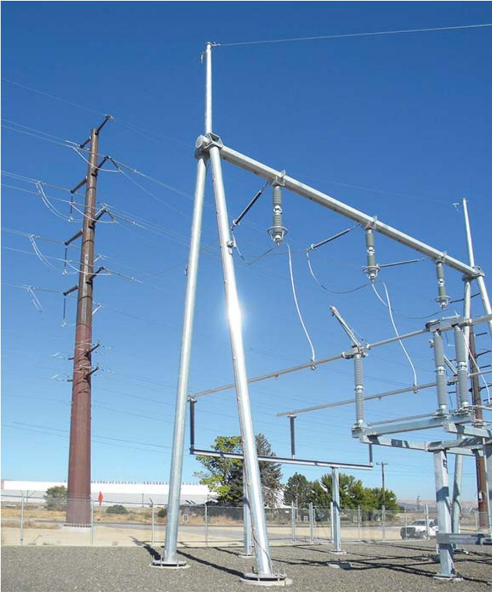
The new Quincy Plains substation includes a 230-kV H-bus rated for 3000 A, a 230-kV live-tank breaker, a 41-MVA 230 x 115/13.8-kV transformer and an eight-bay distribution structure. The new Quincy Plains 230-kV tap will connect the area's new or expanded substations.
