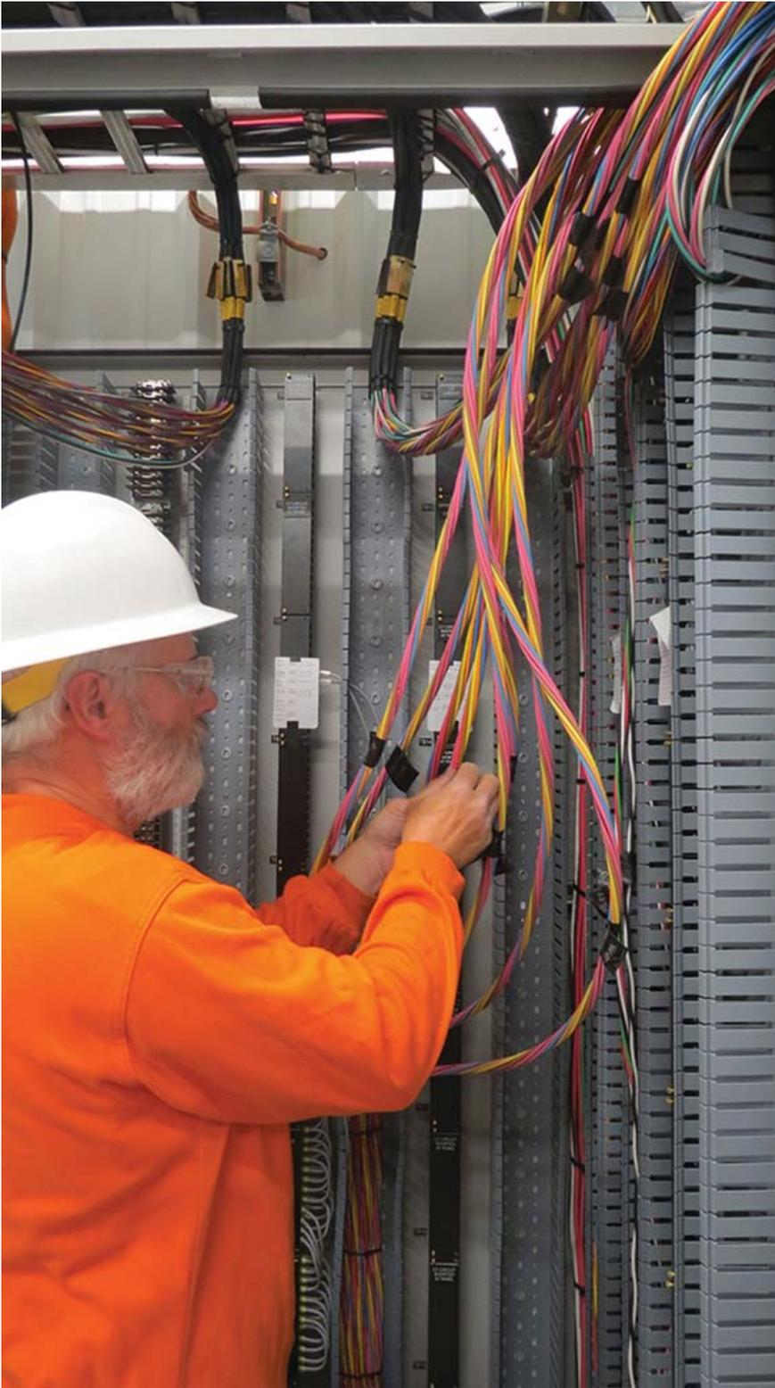
Kenneth Hamelin, foreman for Wilson Construction, in the midst of a 12-day project to wire the marshalling cabinet at Quincy's Cloud View substation.
