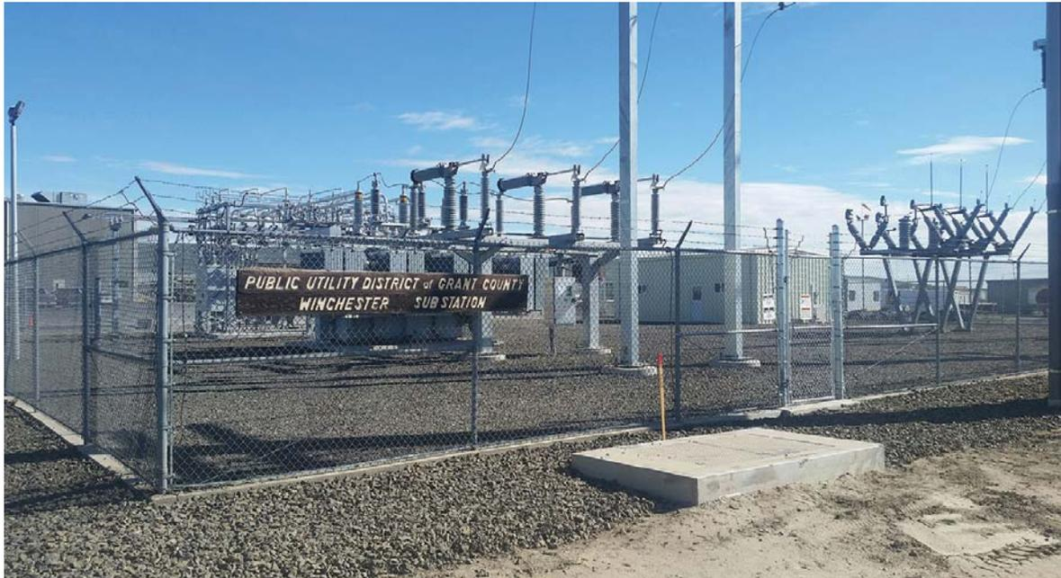
Updated with new equipment that includes a 115-kV circuit switcher and 25-MVA, 115/13.8-kV transformer, with new and reused distribution breakers, the Winchester substation is now ready for future area residential, commercial and industrial growth.
